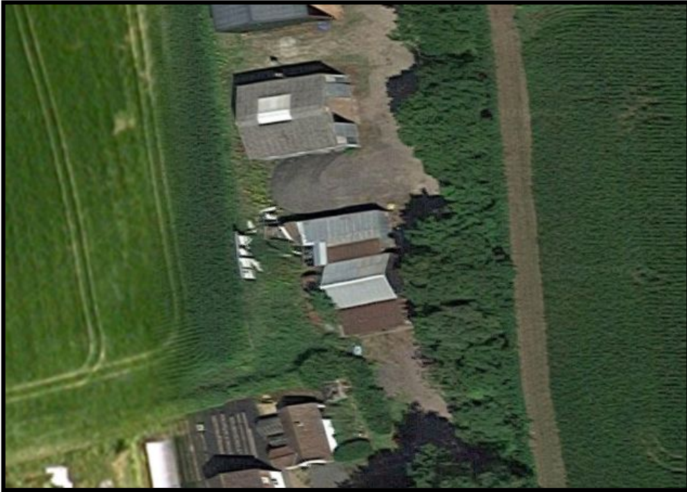
Aerial view of site (Screenshot from Google maps)
