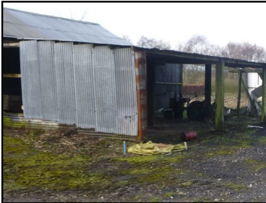
Existing structure (north)
