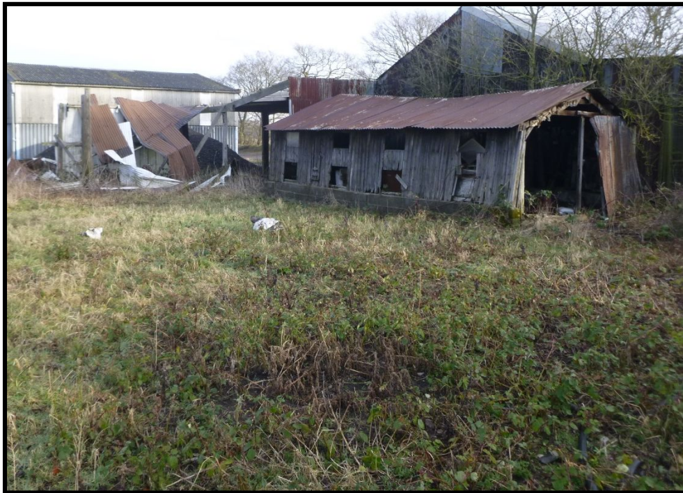
Green area to the west of existing structure
