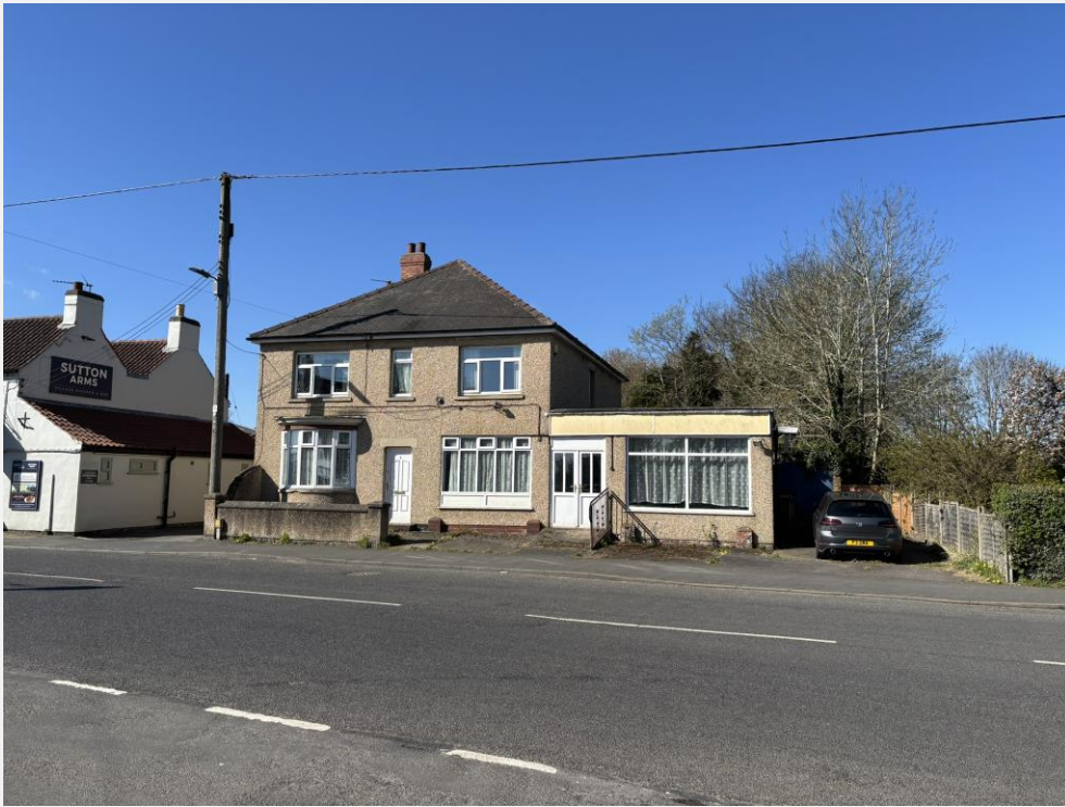
View of East Elevation, Looking West.
