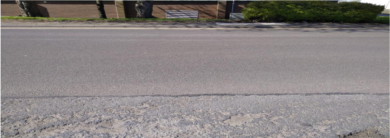
Plate 2.1 – The road, which will connect to the cycle track.
