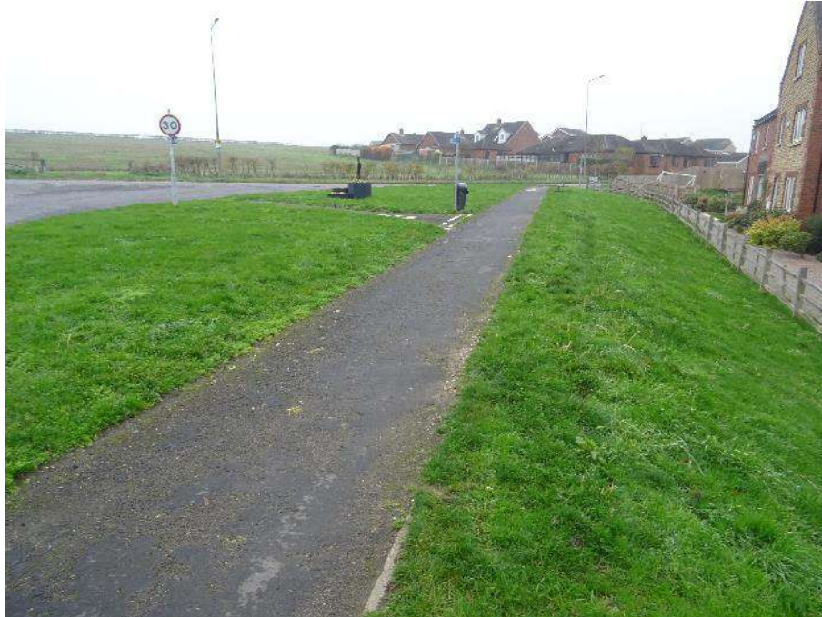
Photo 3: Footway on the Northern Side of the A1077
