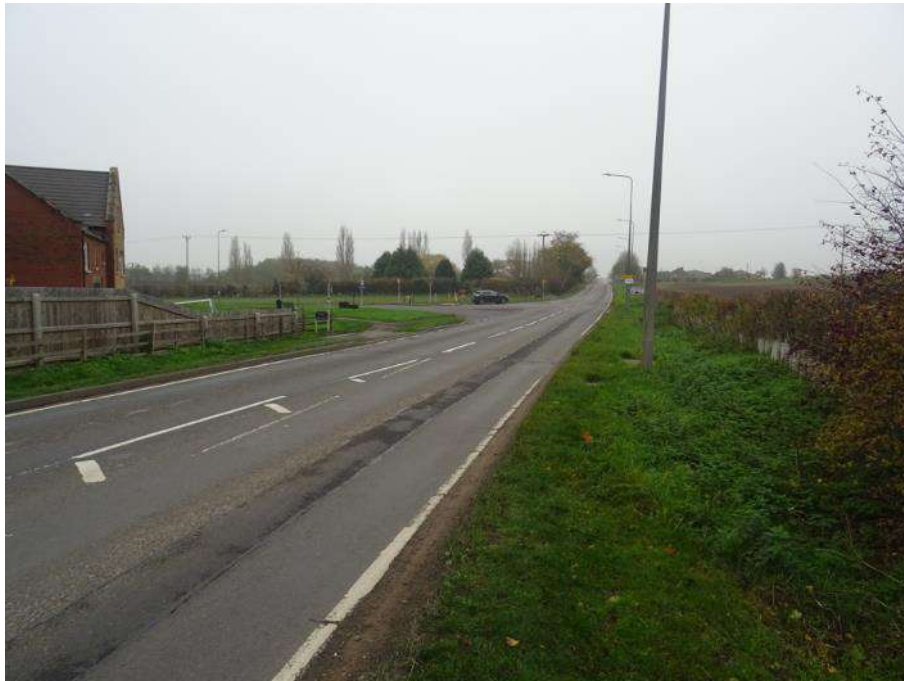
Photo 1: A1077 Along the Site Frontage
