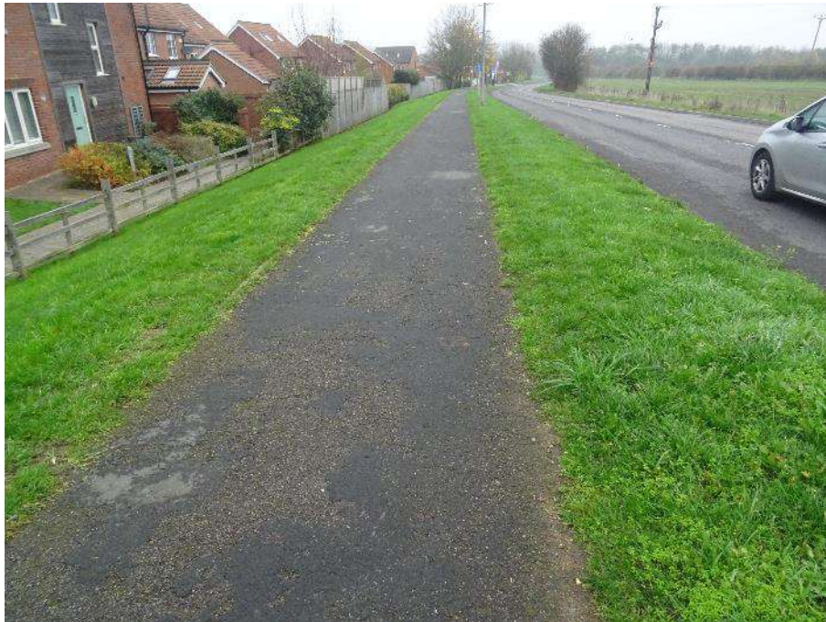
Photo 4: Shared Foot/Cycleway on Falkland Way
