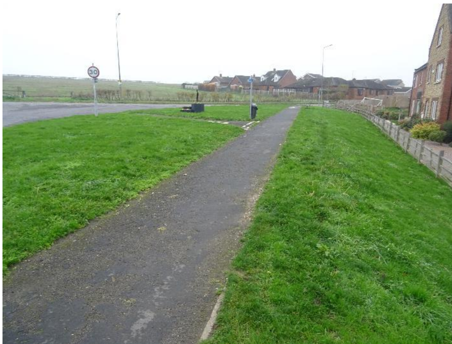
Photo 1: Footway on the Northern Side of the A1077
