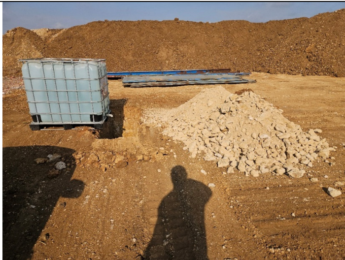
Trial pit TP1 – Excavated spoil
