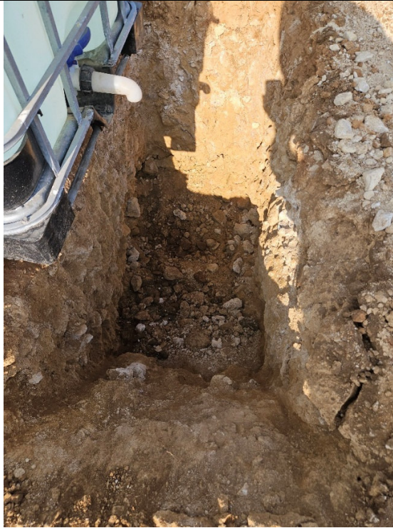
Trial Pit TP1 – After excavations
