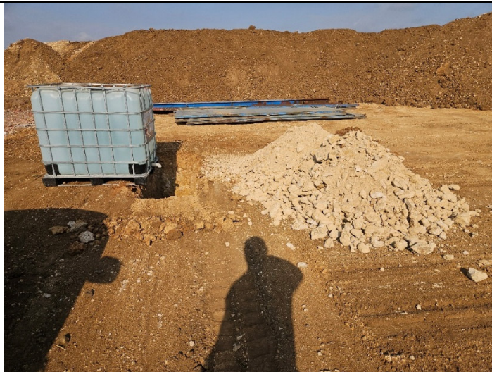
Trial pit TP1 – Excavated spoil
