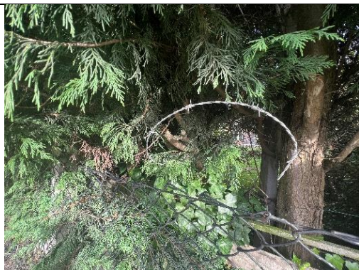
Figure: 6 Sharp barbed wire used as a temporary patch repair by site neighbours – H&S risk
