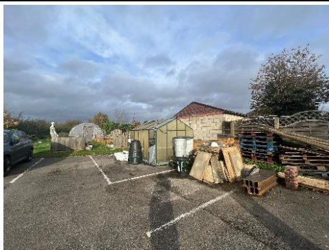
Figure: 11 General view of unsecured east boundary – H&S risk
