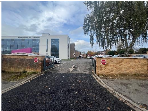
Figure: 15 Entrance gate provides inadequate security to school – H&S risk
