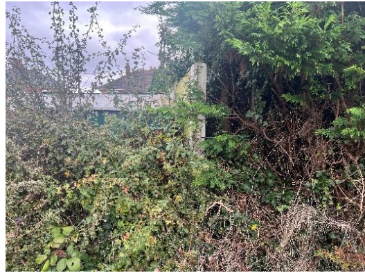
Figure: 2 Large hole in site boundary – H&S risk
