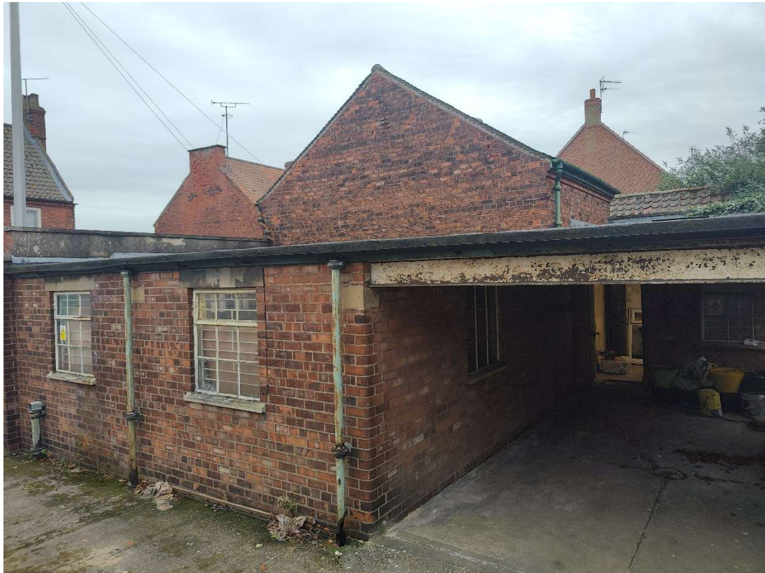
Figure 9 (Flat Felt Roof).
