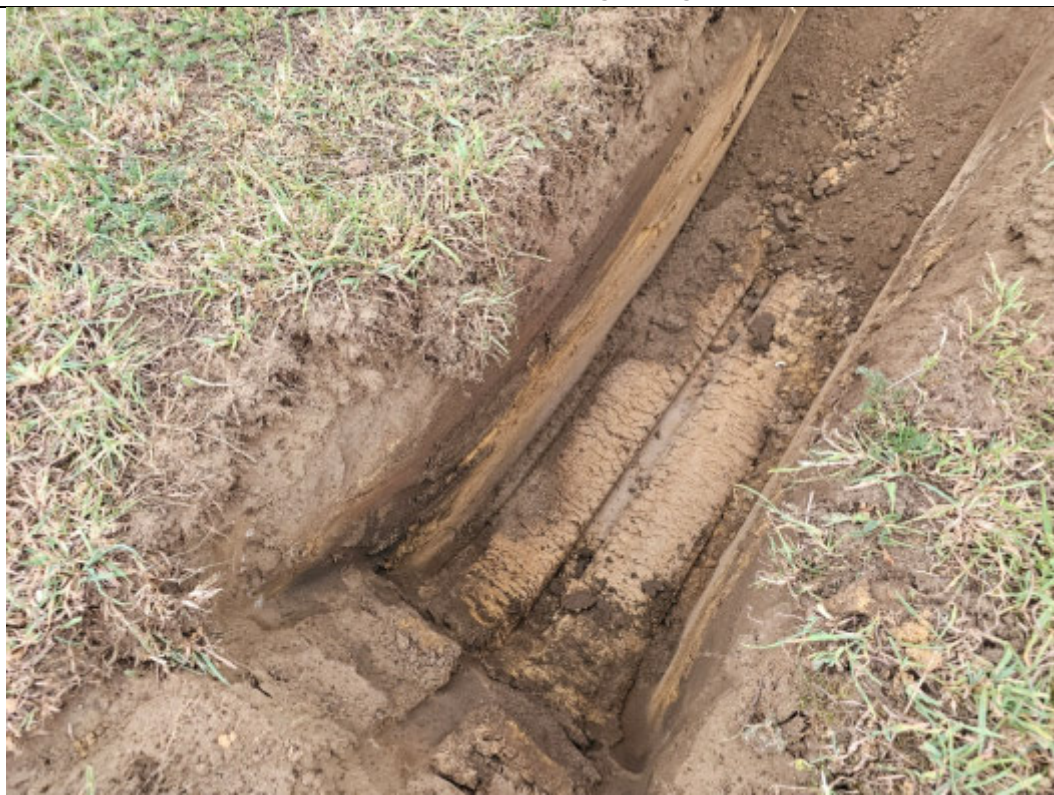
Trial Pit TP2 - After excavations
