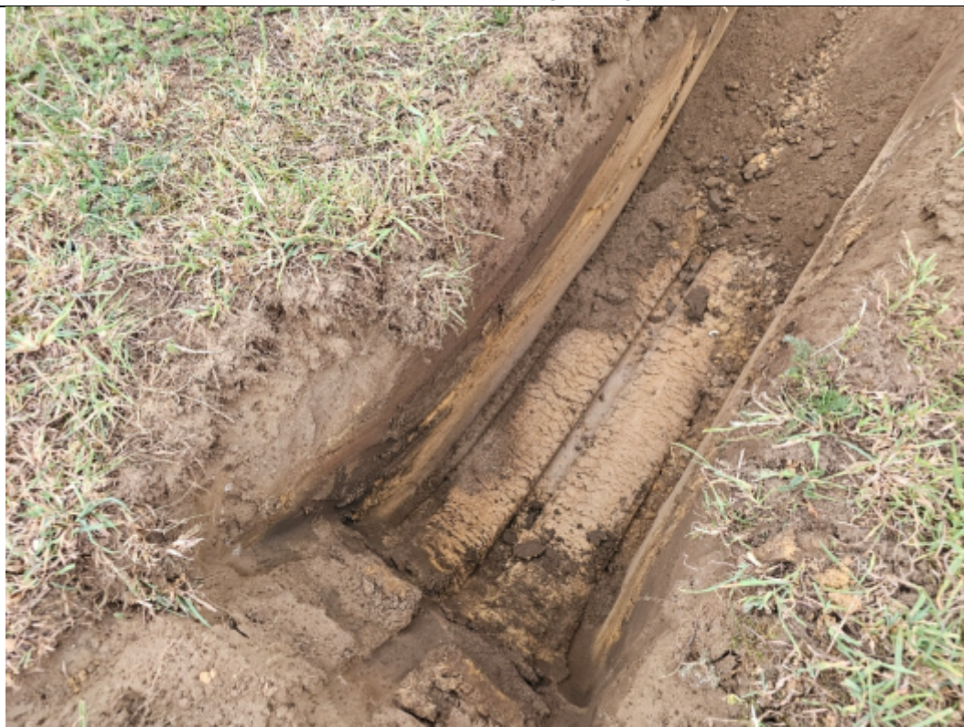
Trial Pit TP2 - After excavations
