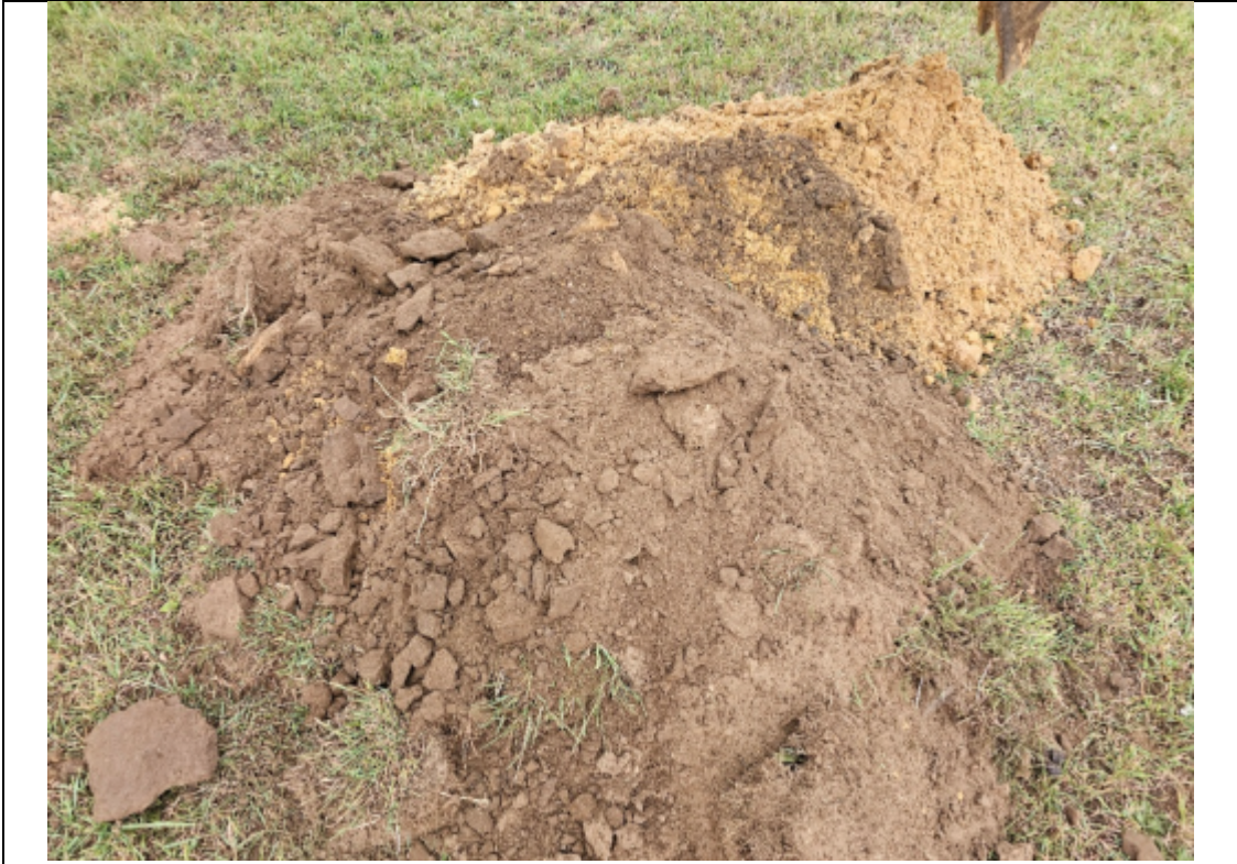
Trial pit TP2 - Excavated spoil
