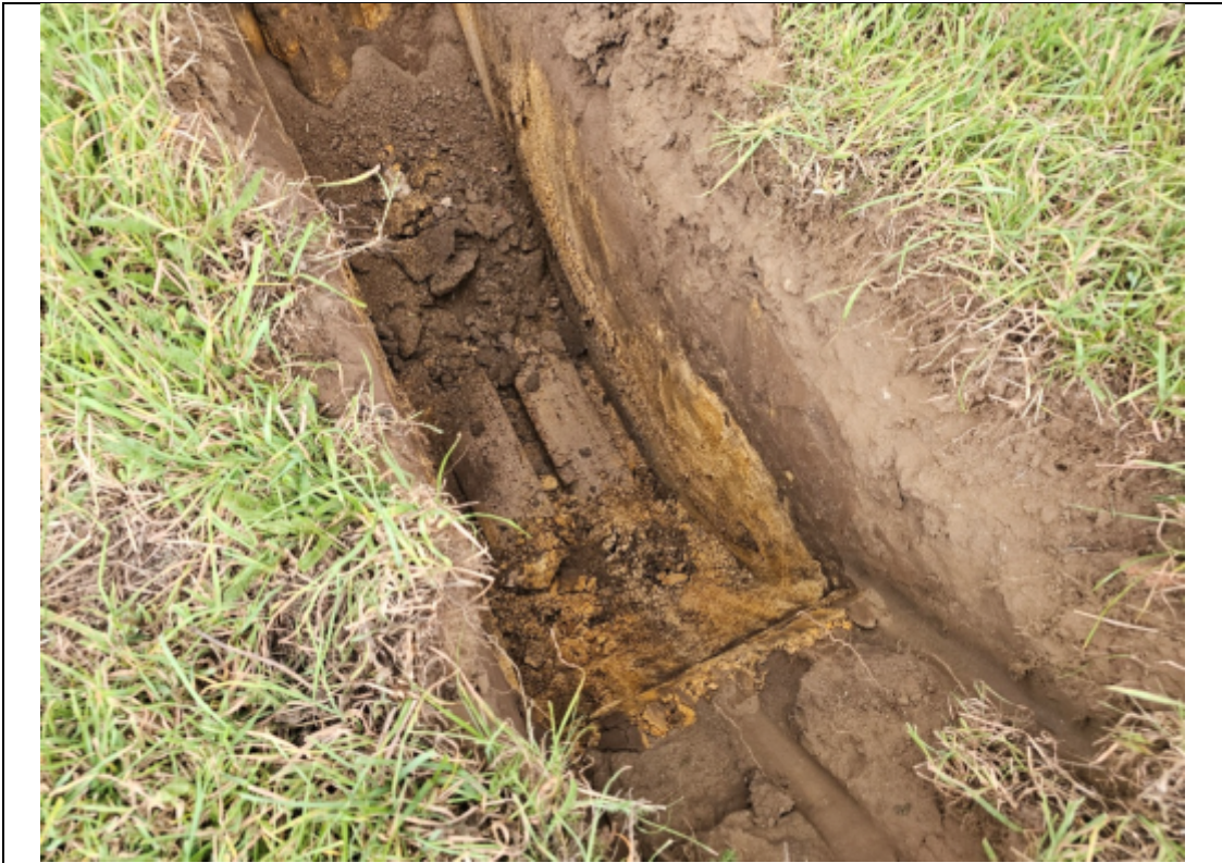
Trial Pit TP1 - After excavations
