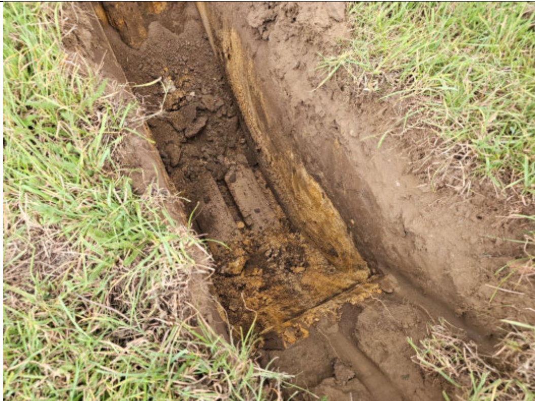
Trial Pit TP1 – After excavations
