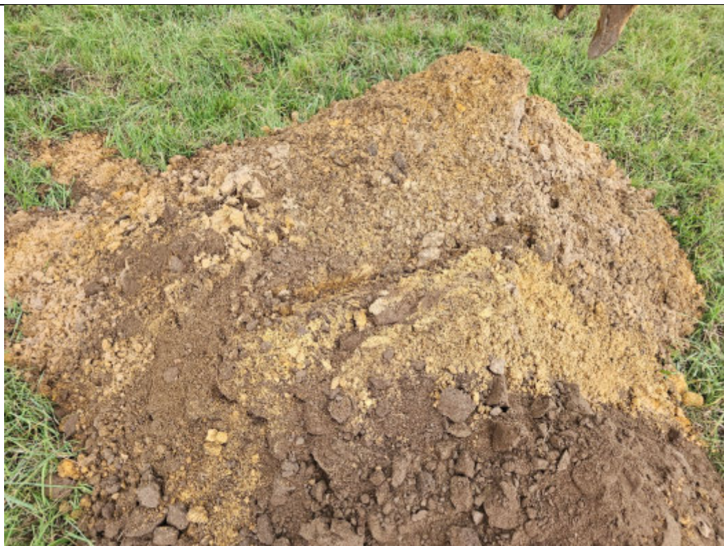
Trial pit TP1 – Excavated spoil
