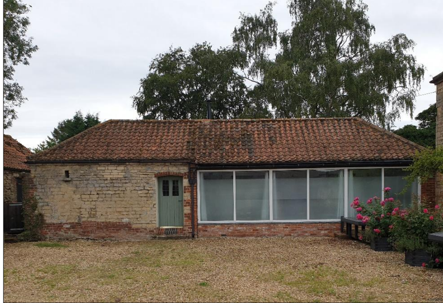
Photograph 1: The property at Swallows Nest, eastern elevation
