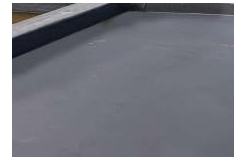
Membrane Finish Flat Roof
