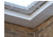
White UPVC Fascia to match existing
