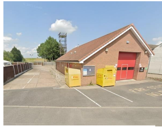
Existing Fire Station showing access to parking down the west elevation
