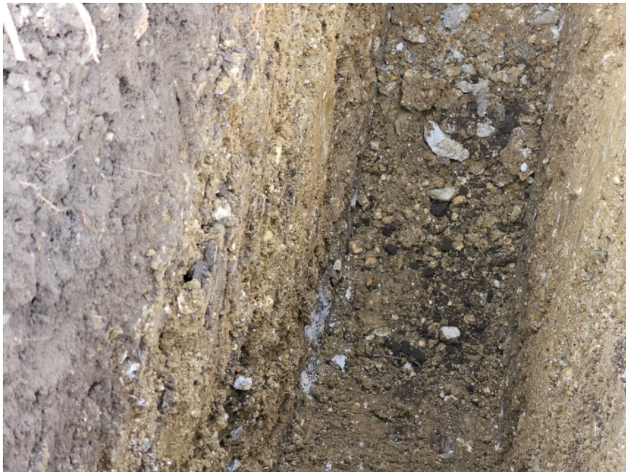
Site investigation photo: 6 Photo direction: - Description: TP202
