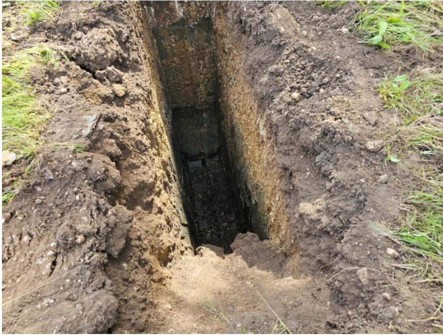
Site investigation photo: 15 Photo direction: - Description: TP205
