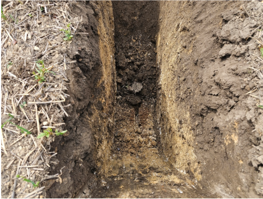
Site investigation photo: 25 Photo direction: - Description: TP208
