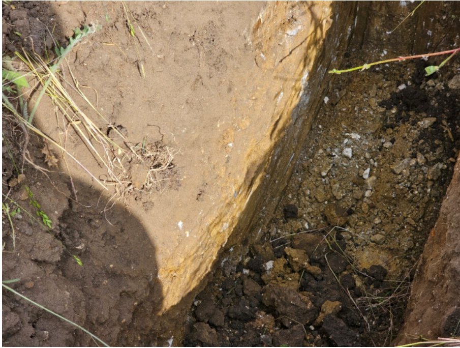
Site investigation photo: 13 Photo direction: - Description: TP204
