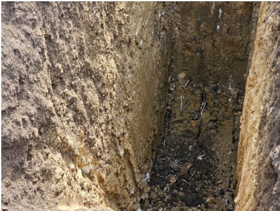
Site investigation photo: 2 Photo direction: - Description: TP201
