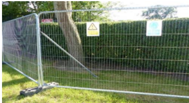
Example of Tree Protection measures if required
