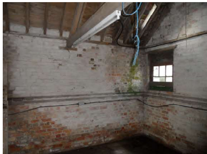
Plate 28 North eastern corner of Room 3.
