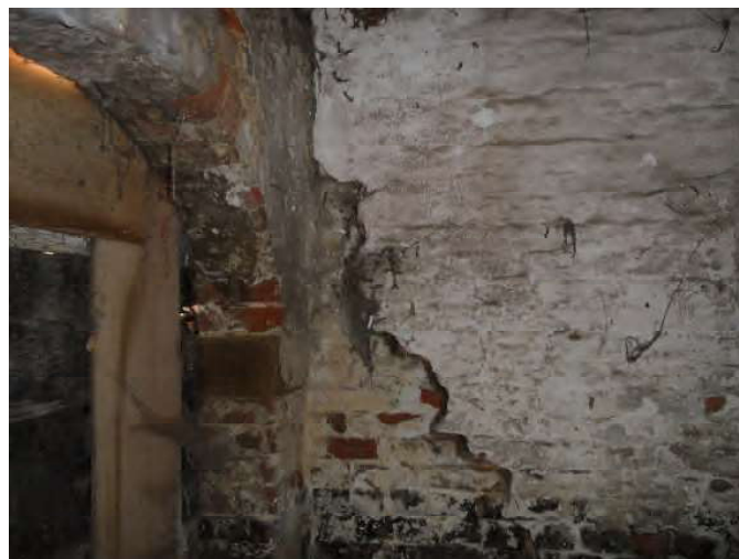
Plate 20 Eastern wall within the ground floor Garage area.
