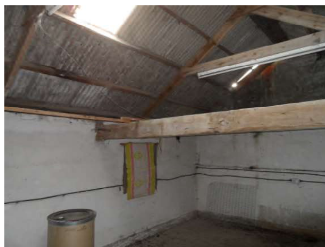
Plate 24 Roof construction over the first floor of the Main Barn.
