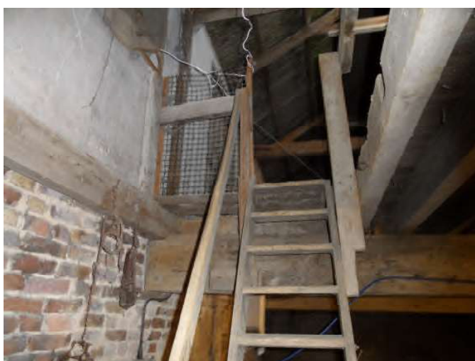
Plate 23 Ship ladder access to the first floor storage area.
