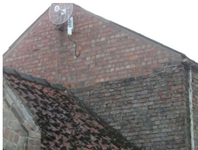
Plate 6 Eastern elevation of the Main Barn (First floor level).
