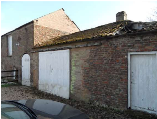
Plate 1 Northern elevation of the barn complex (western side).
