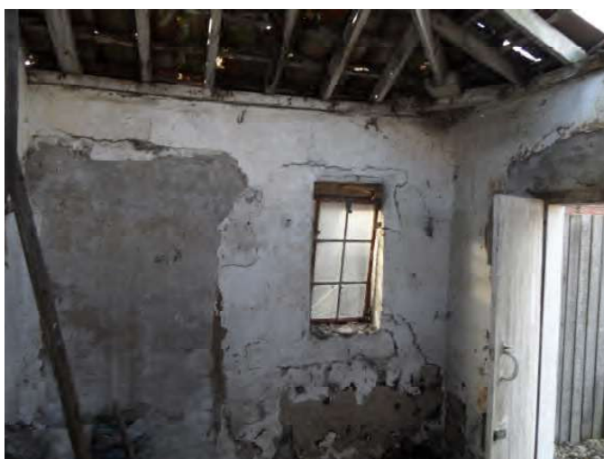
Plate 17 North eastern corner of Room 2.
