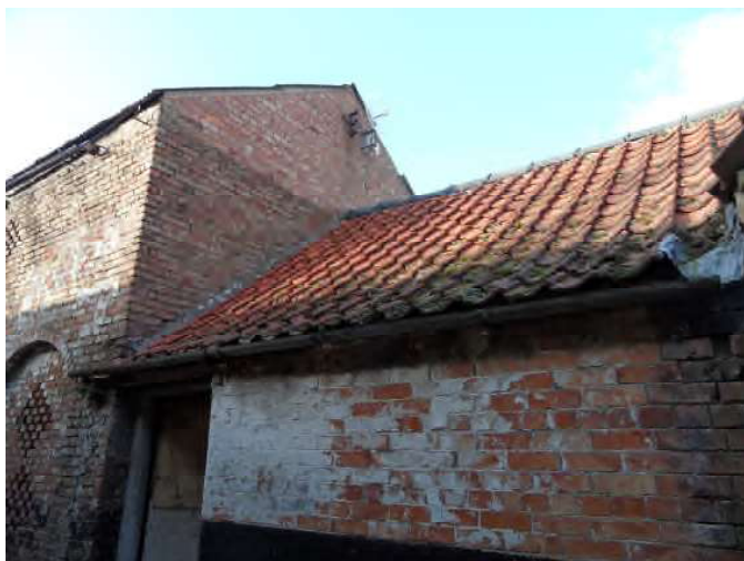
Plate 9 South eastern corner of the Main Barn.
