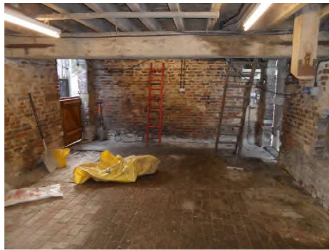
Plate 22 Main ground floor barn area (looking east).
