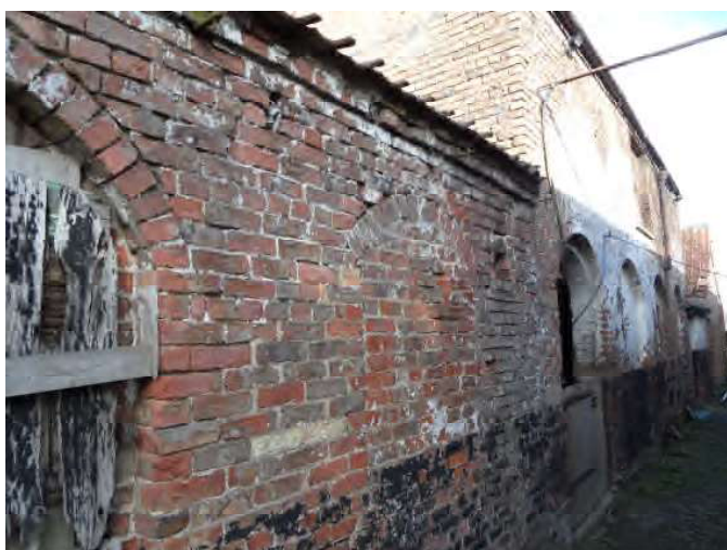
Plate 11 Plate 8 South elevation of the building complex (western end).
