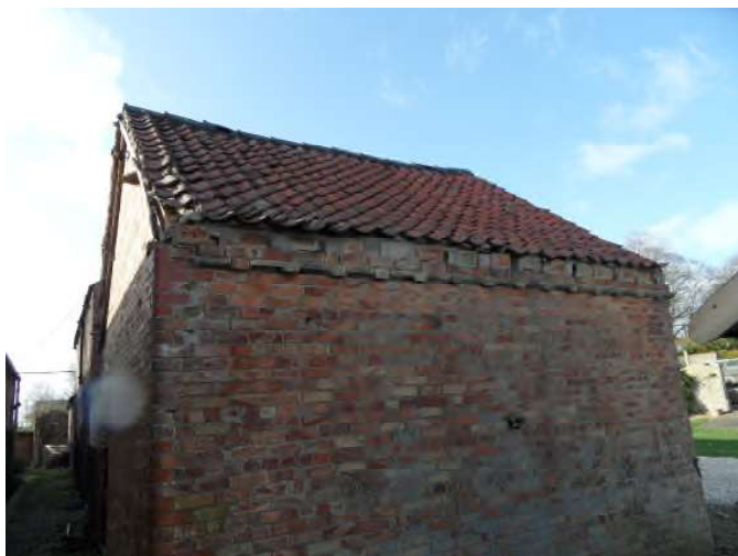
Plate 7 Eastern elevation of the building (forming Room 3).
