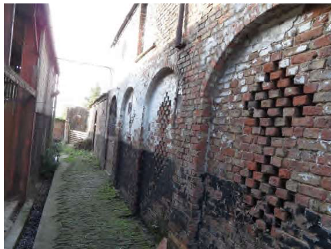
Plate 10 Feature arches on the south elevation of the Main Barn.
