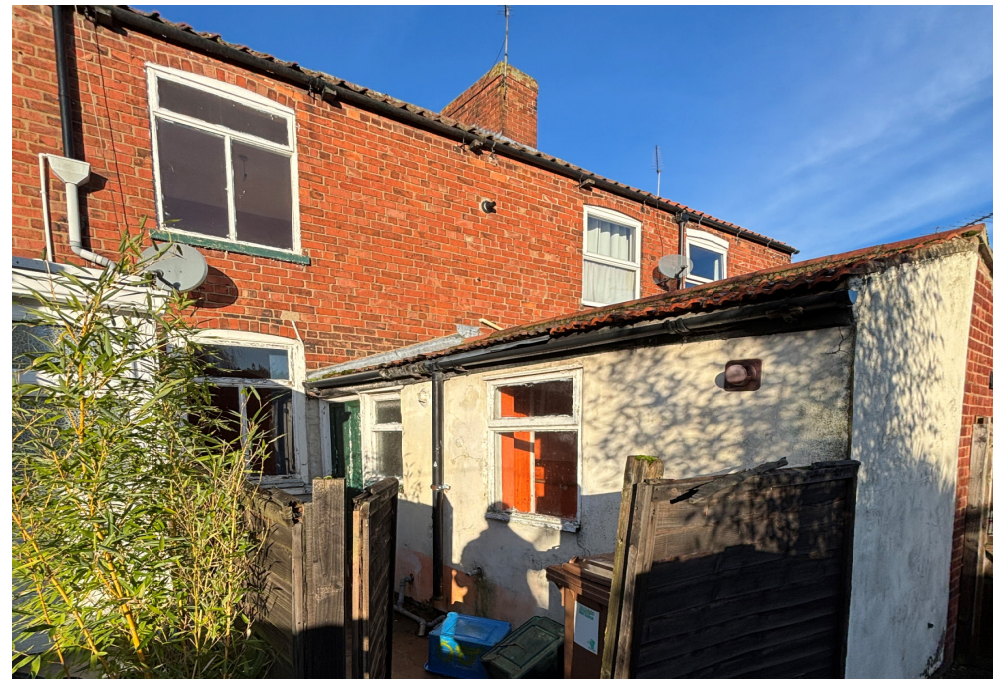
View looking East at the existing rear extension.
