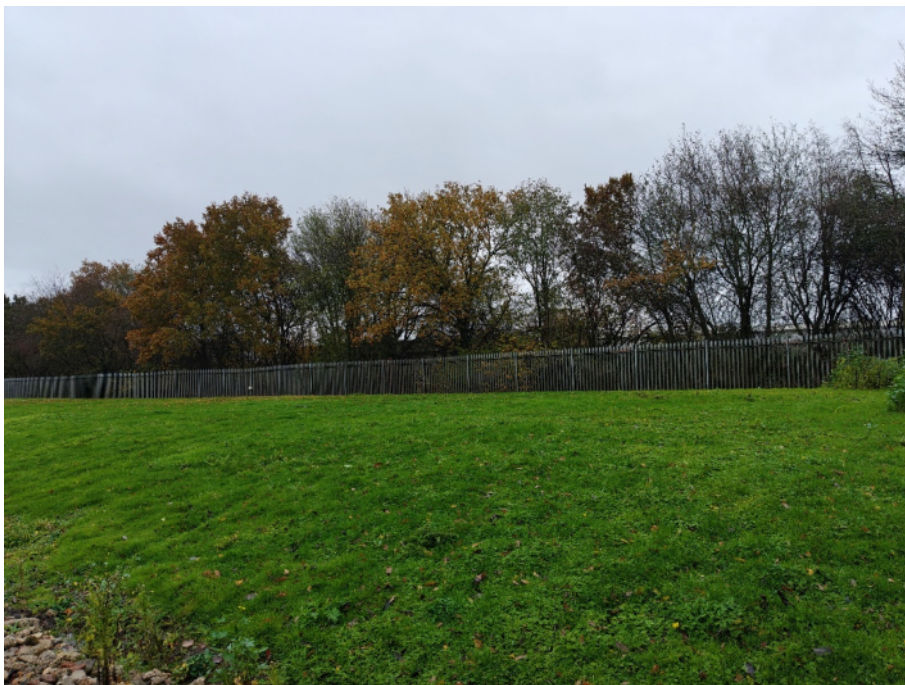
Site walkover photo: 15 Date: 11 Nov 2025 Photo direction: Southeast Description: Grassy embankment (c. 0.7m-high)
