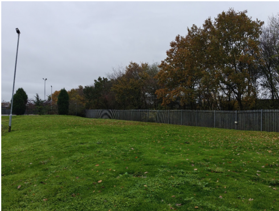
Site walkover photo: 19 Date: 11 Nov 2025 Photo direction: East Description: Grassy embankment (c. 0.7m-high)
