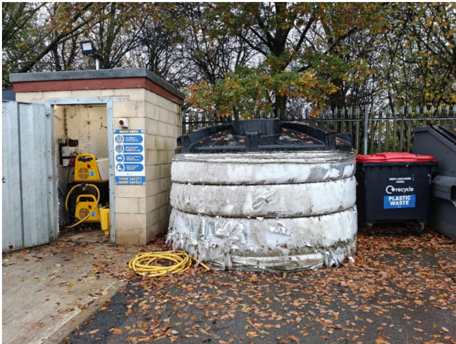
Site walkover photo: 13 Date: 11 Nov 2025 Photo direction: West Description: Large, insulated water tank next to pump house for the vehicle washdown area
