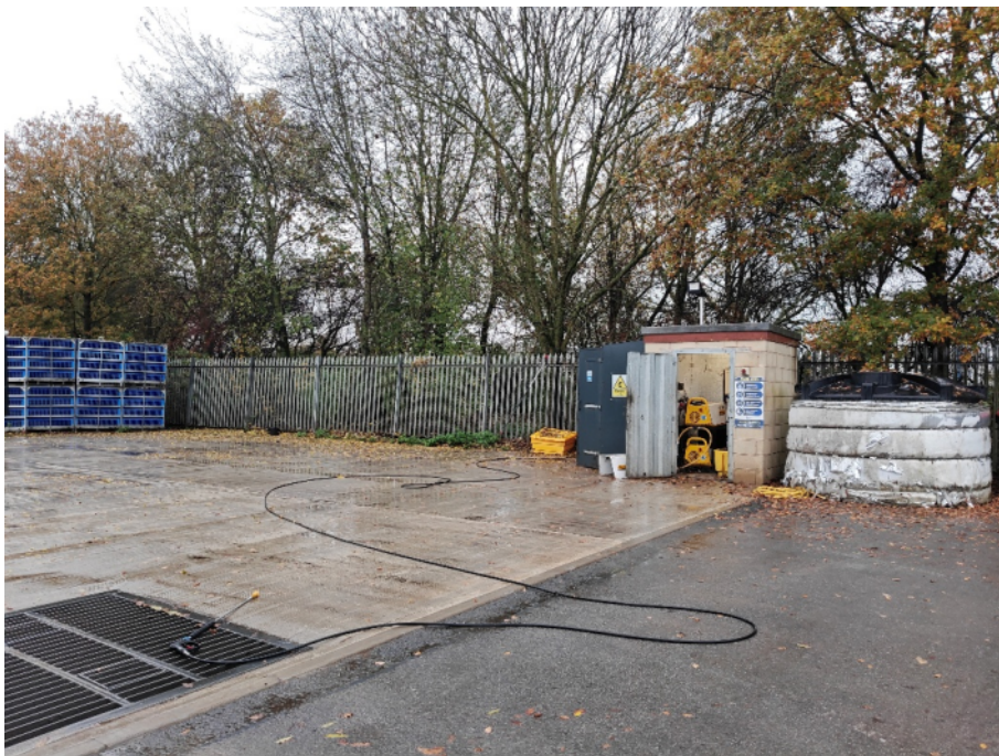
Site walkover photo: 11 Date: 11 Nov 2025 Photo direction: South Description: Concrete washdown area with drains and poultry crates (left)
