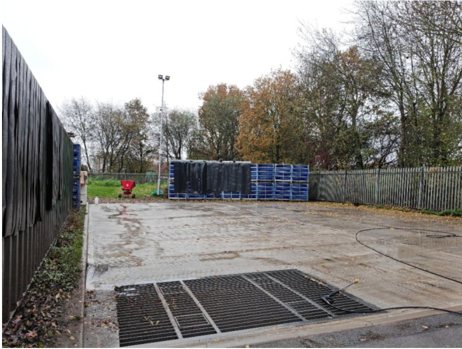
Site walkover photo: 12 Date: 11 Nov 2025 Photo direction: South Description: Concrete washdown area with drains and poultry crates
