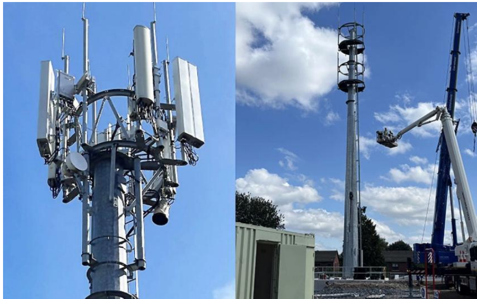
Image 2b: Example of a monopole with open headframe (Source: FLI)
