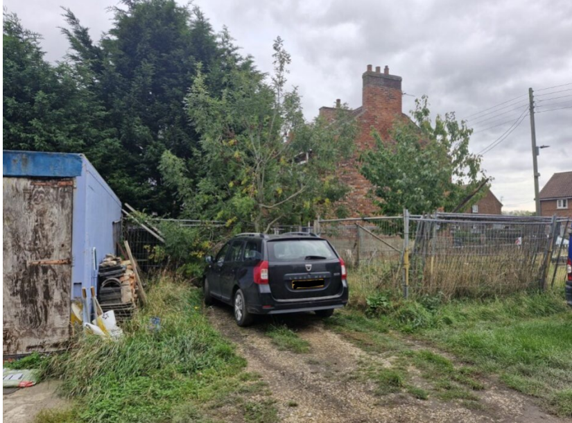
Figure 6: Application site from Manchester Square
