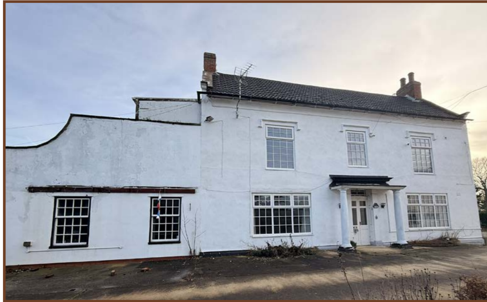
Plate 1 - Main (west) elevation
