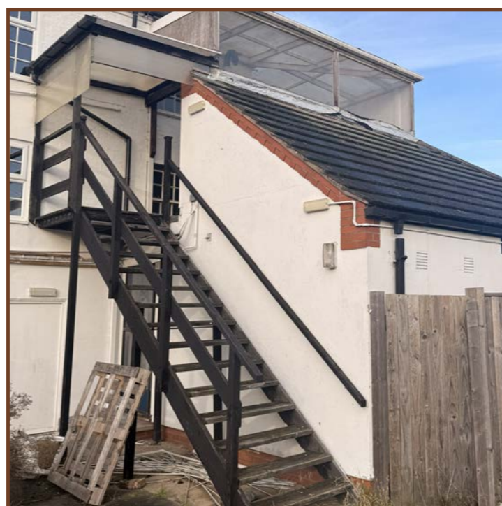
Figure 26 - Timber stair access to decking/landing area.
