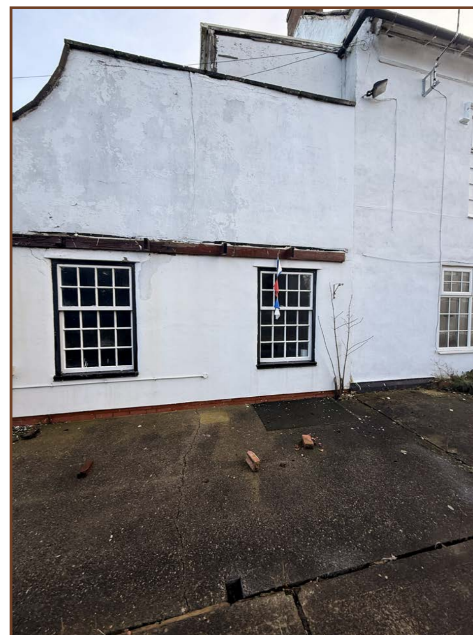
Figure 27 - View of canopy above screen wall.
