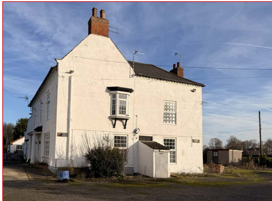
Figure 2 - View of southern elevation.
