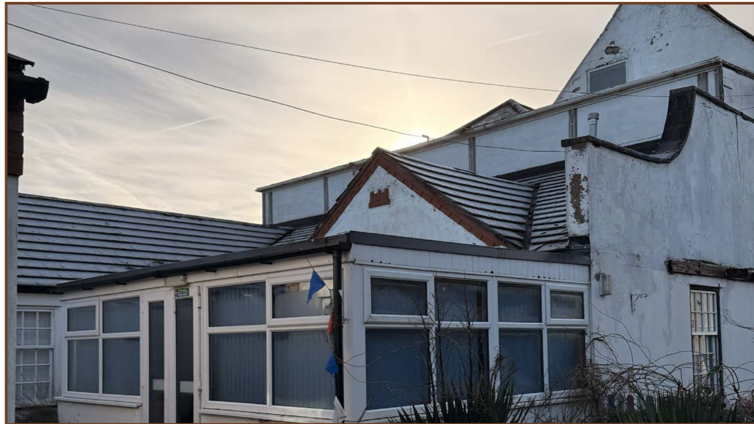
Plate 4 - Side (northern) elevation.
