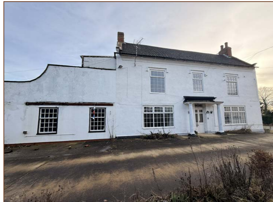
Figure 3 - View of western (principal) elevation.
