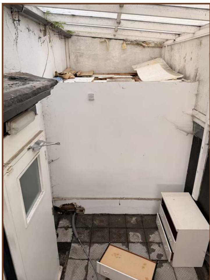
Figure 24 - Bathroom to be demolished.
