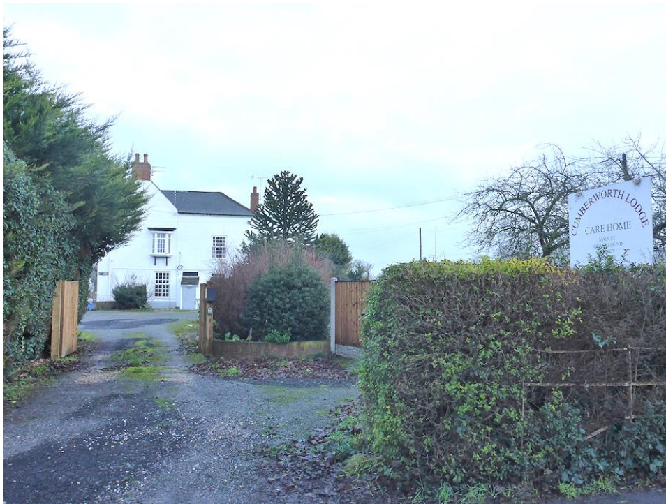
Cumberworth Lodge looking north from Main Street.
