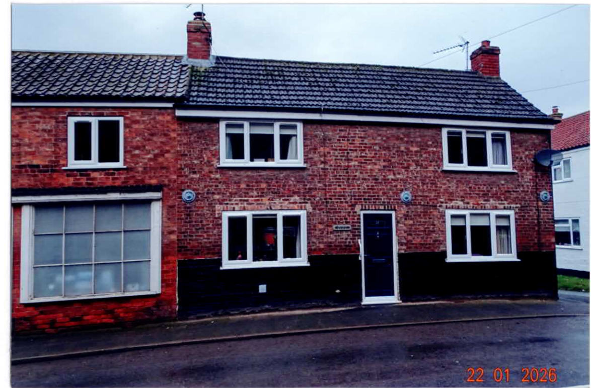
SHOP CONVERSION – Facing South East
