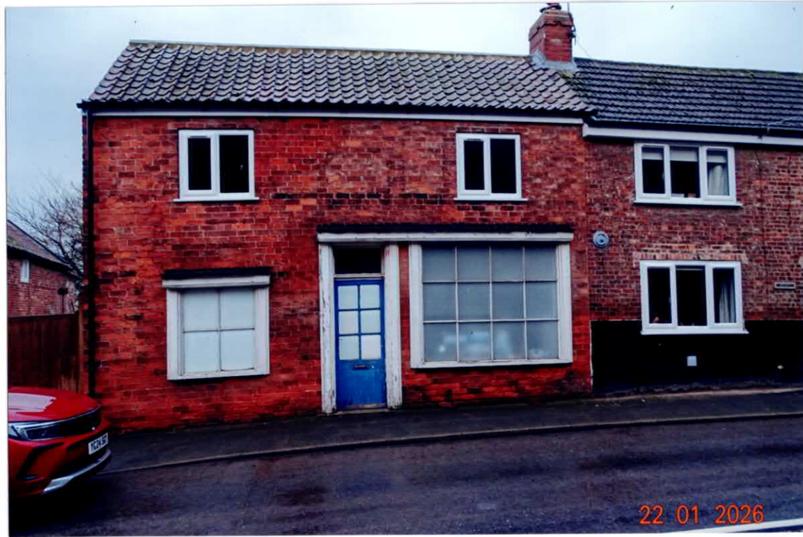
SHOP CONVERSION – Facing South East
