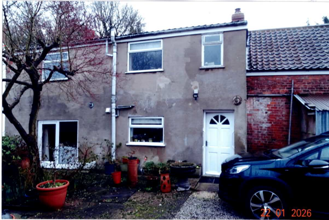
SHOP CONVERSION – Facing North West
