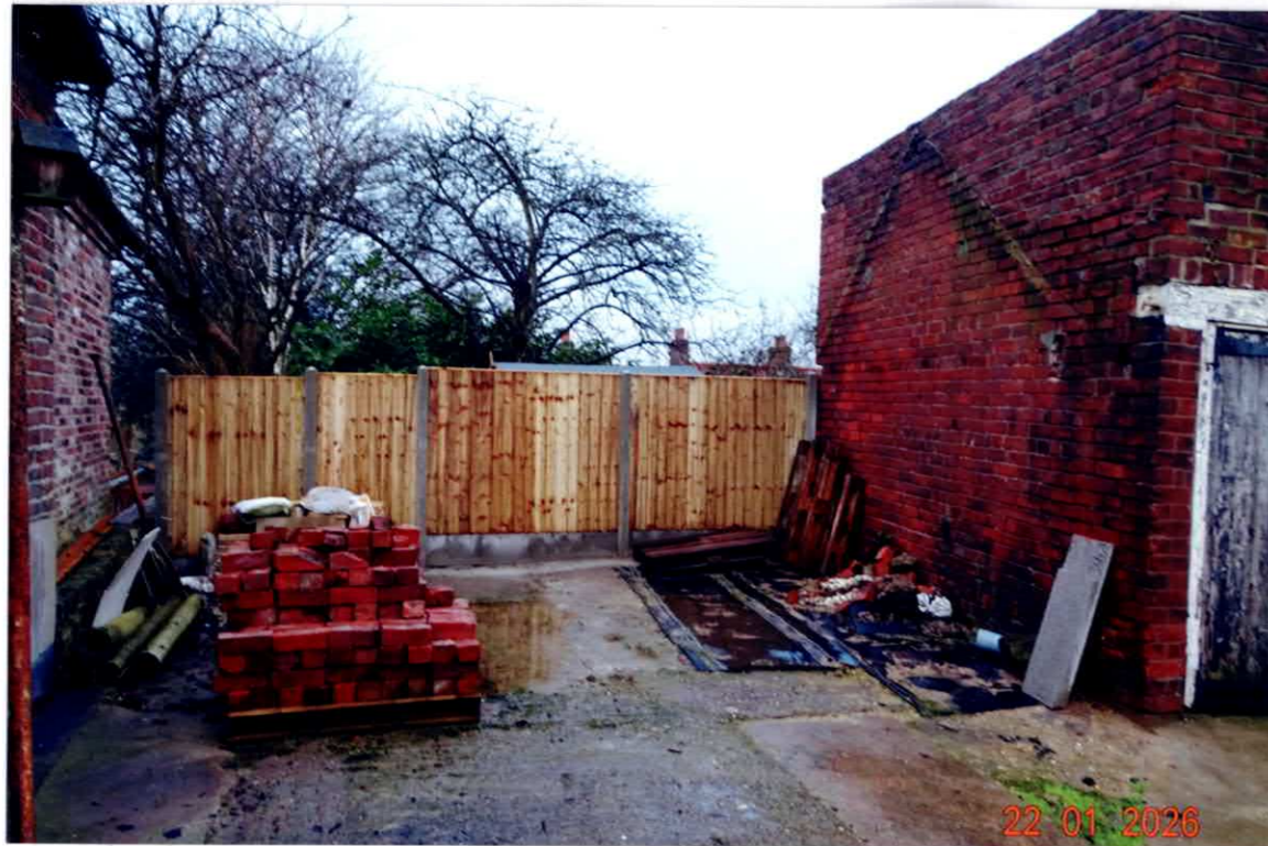
GARAGE CONVERSION – Facing South West
