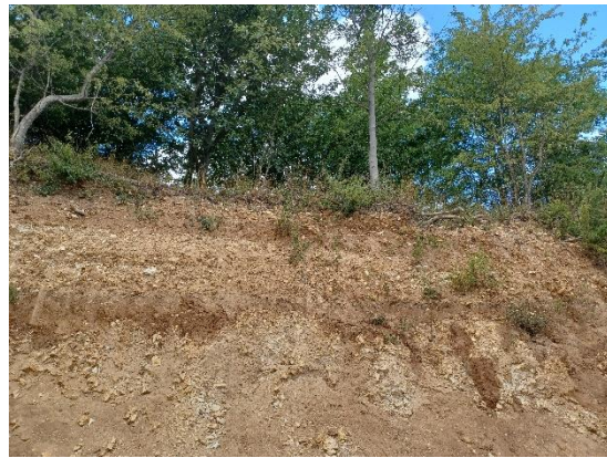
Photograph 19: trees and scrub on southern rail embankment
