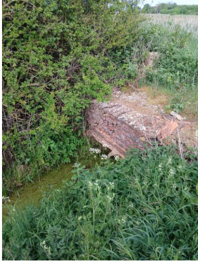
PHOTO 9 CULVERT TN1 WITH BAT ROOST POTENTIAL
