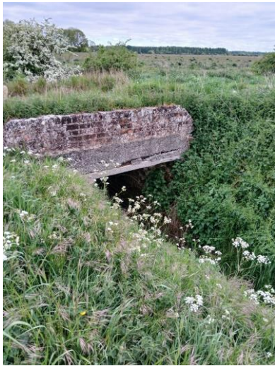
PHOTO 10 CULVERT TN2 WITH BAT ROOST POTENTIAL
