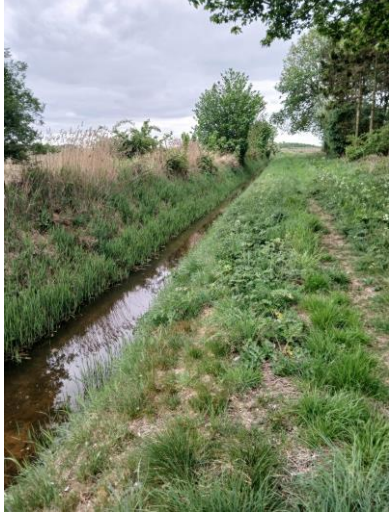
PHOTO 3 WATERCOURSE RW1B (THIRTY FOOT DRAIN LWS)
