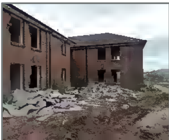
Figure 5. Building 87 following asbestos removal awaiting demolition
