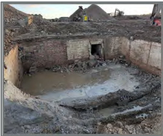
Figure 15. Building 42 bunker exposed
