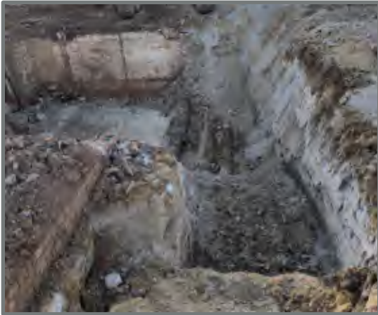
Figure 19. Building 38 bunker exposed
