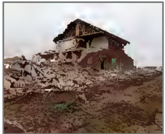
Figure 4. Building 86 demolition in progress following asbestos removal works
