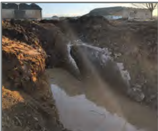
Figure 17. Building 44 bunker exposed, in process of removal
