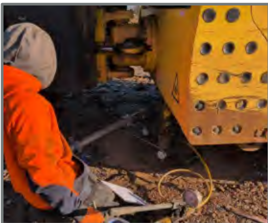
Figure 35. CBR testing on road corridors
