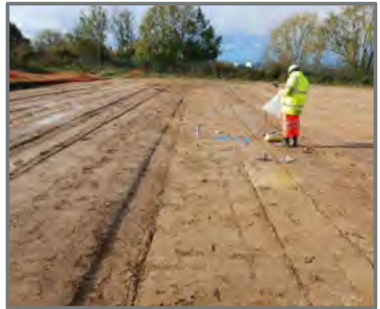
Figure 34. NDT testing on completed turnover area
