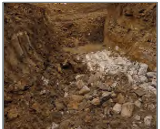
Figure 18. Building 44 bunker excavation
