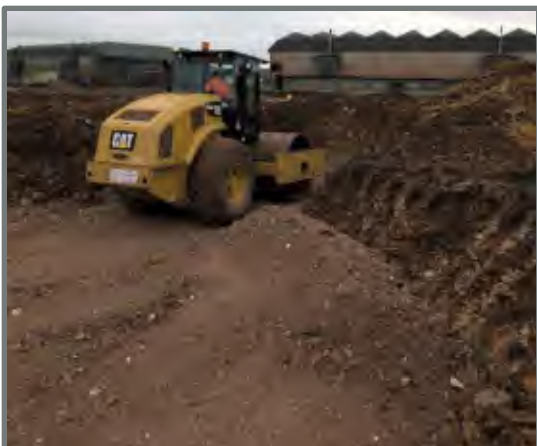
Figure 23. Compaction of reinstated 1A materials into B44 bunker excavation
