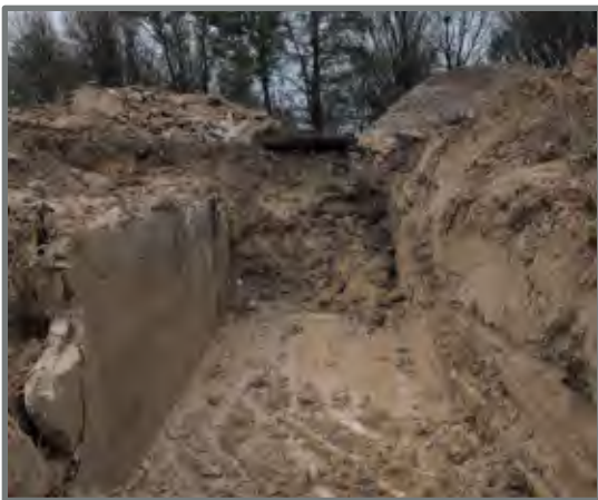
Figure 21. Building 39 bunker excavation
