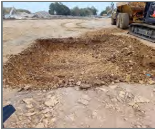
Figure 9. Clean base and sides of hotspot WS03
