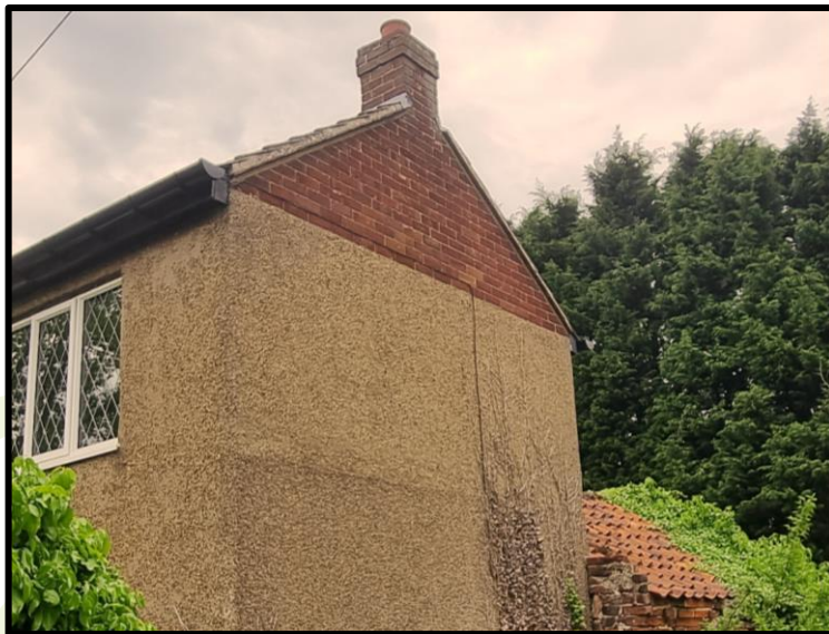
Figure 5: Intact eastern gable.
