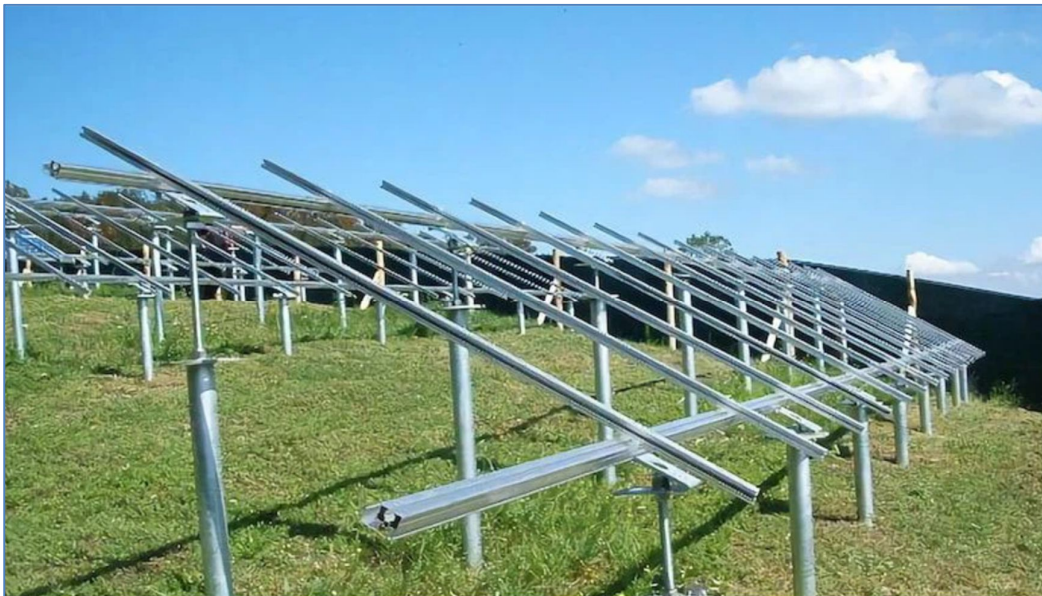
Figure 2 Typical piled supports for solar tables
