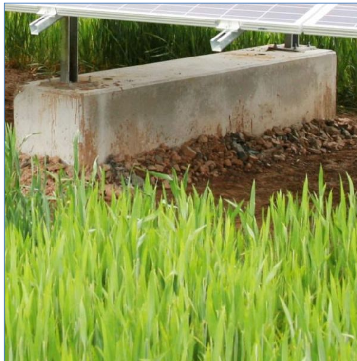
Figure 3 Examples of ground-mounted solutions employed to preserve archaeology in situ
