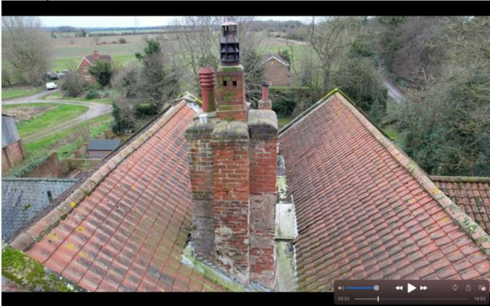
Chimney A – Northern face
