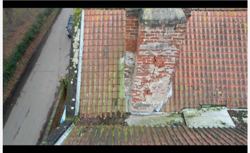
Chimney A – Western face
