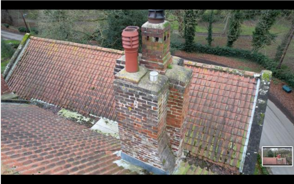
Chimney A – Eastern face
