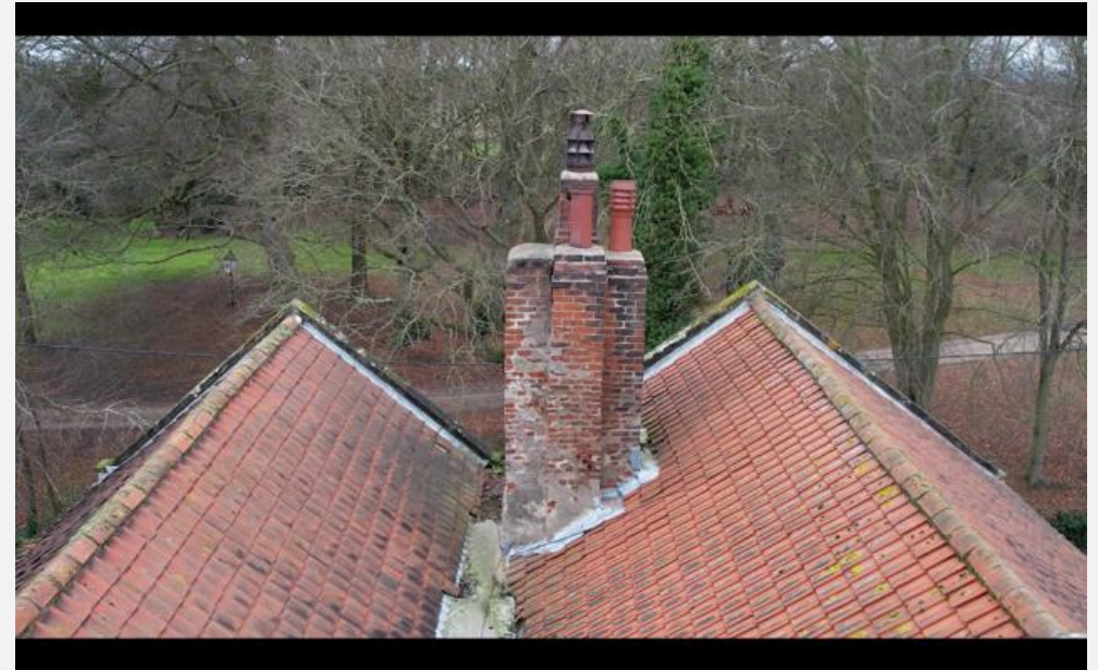
Chimney A – Southern face
