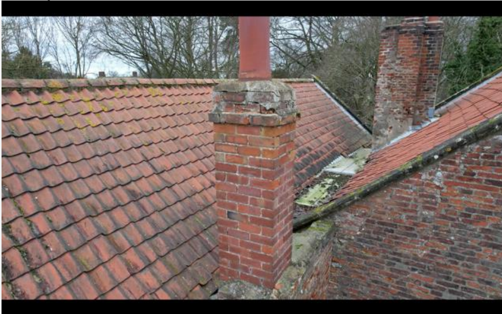
Chimney B – Southern face
