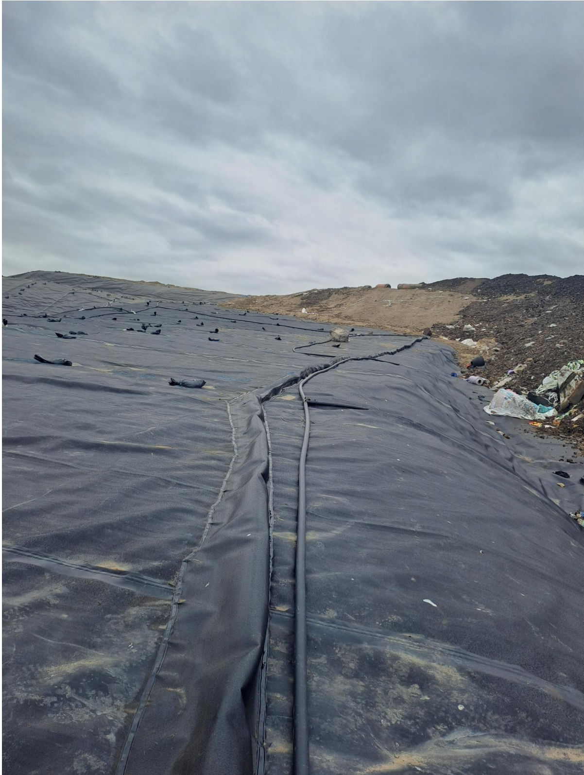
Photo 4: Taken from the north west of the site looking south.
