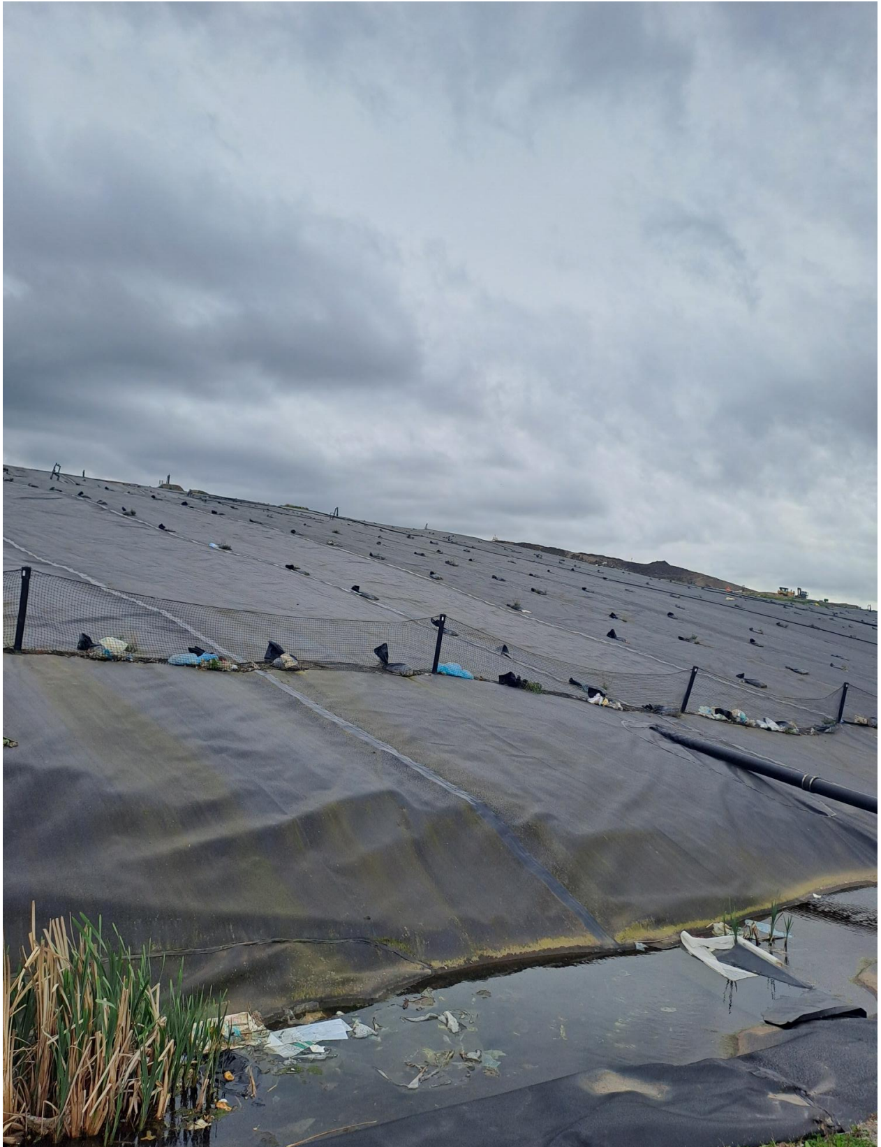
Photo 6: Taken from the north west of the site, looking south east
