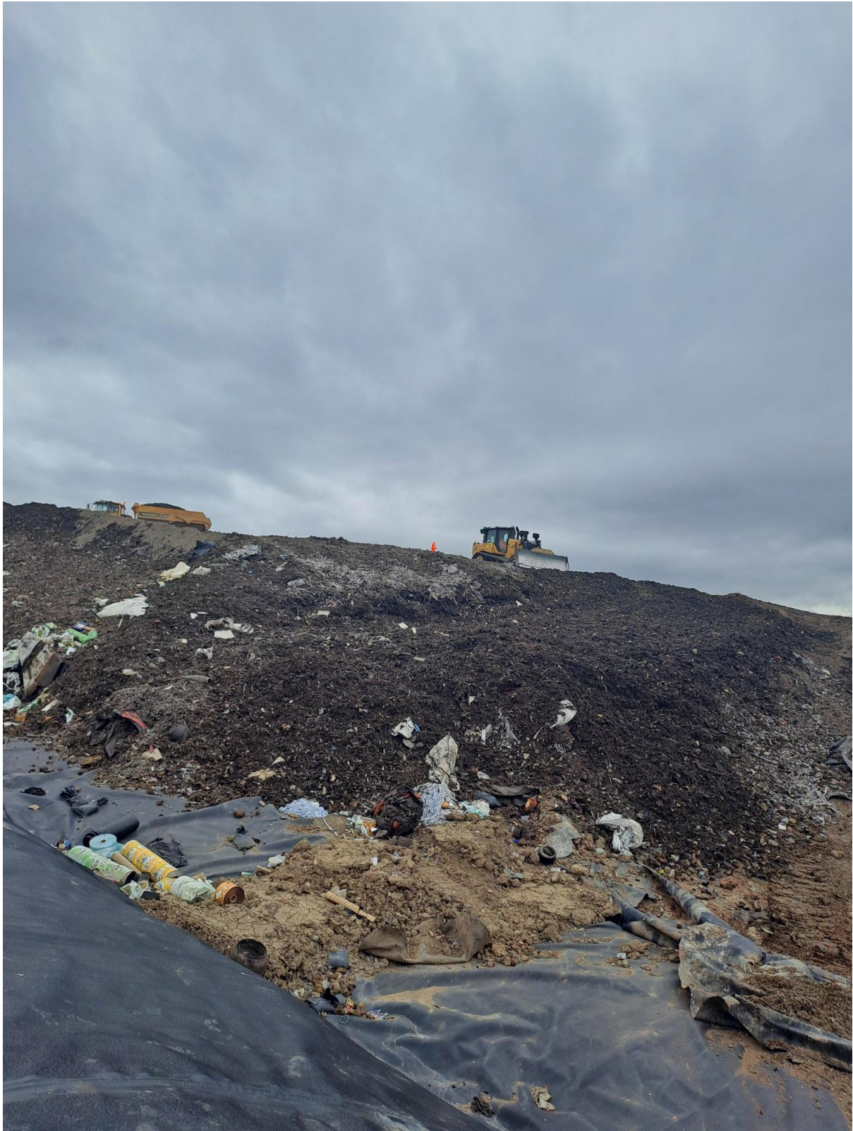
Photo 3: In the north of the site, looking west to where infilling is taking place.
