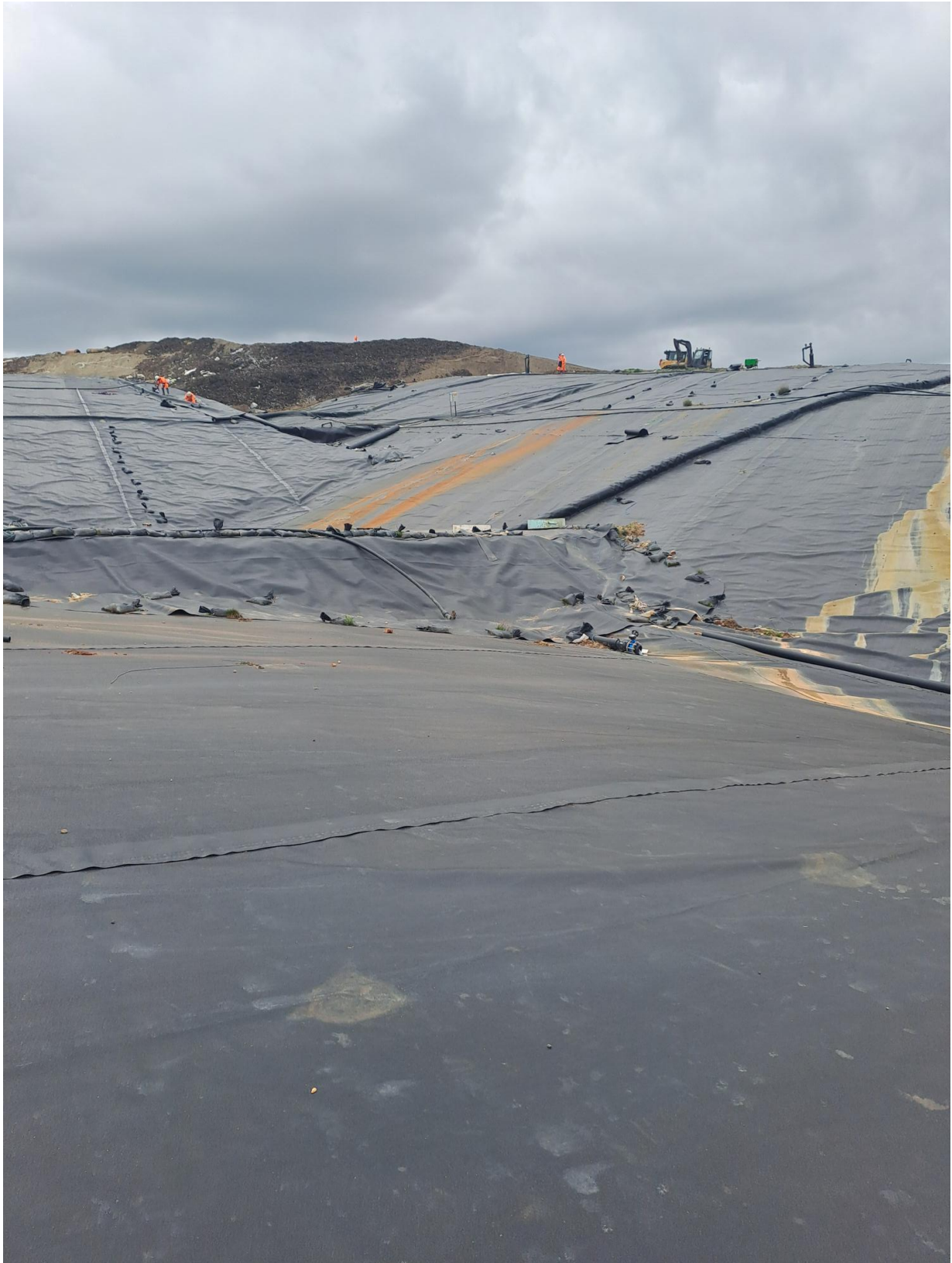
Photo 5: Taken from the north west of the site, looking south
