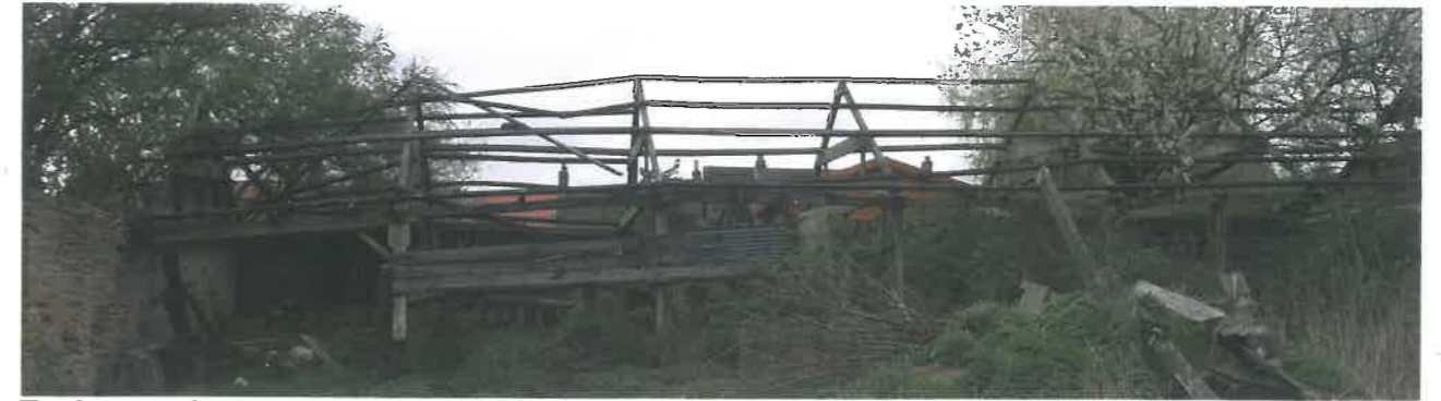
The framework of the former farm buildings
