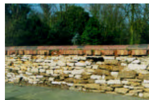
◀ Appleby-dry stone wall with brick and tile coping. Softness of stone is leading to erosion and may result in wall collapse if not repaired.
