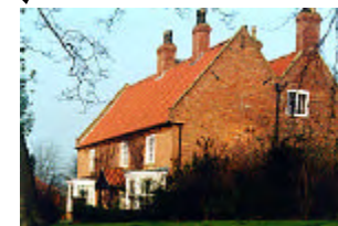
▲ Larger Wolds house illustrating traditional brick and pantile construction, steep roof pitch, tumbling in and stone coping at gable ends
