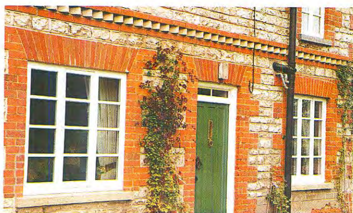
Typical building detail on an Estate cottage.
