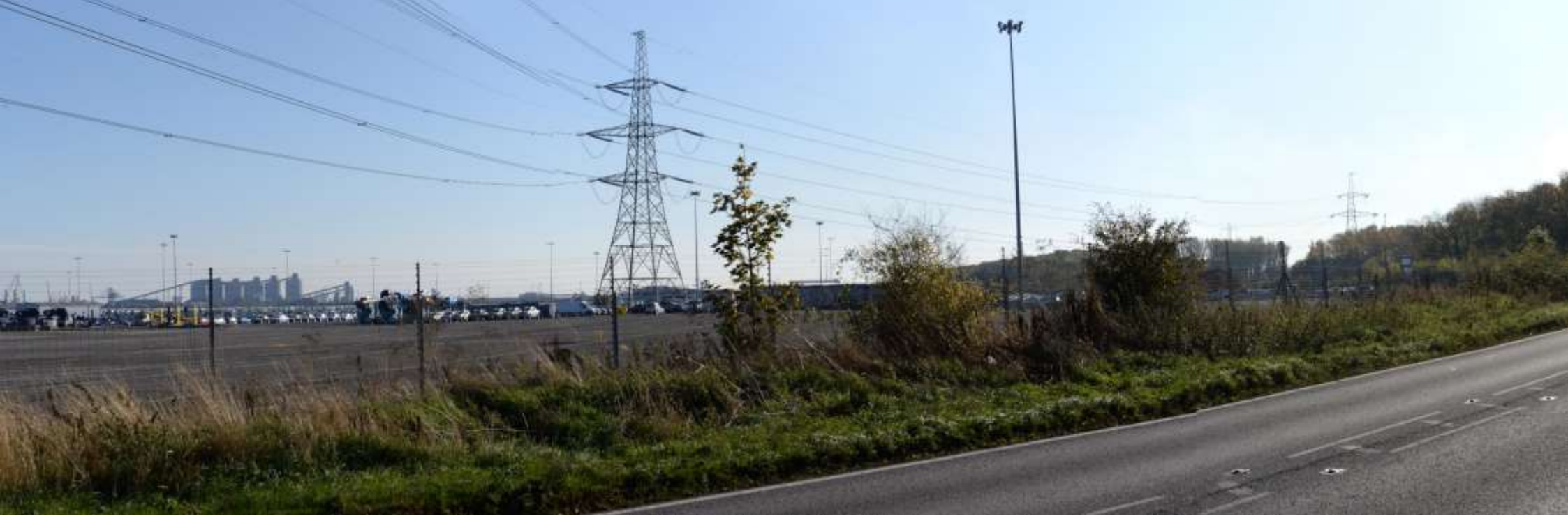
Figure 68 – View south from Haven Road
