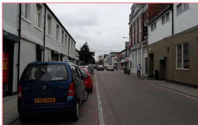
Above: The use of different materials on this street in Scunthorpe defines the parking provision and visually narrows the carriageway, encouraging slower speeds.
