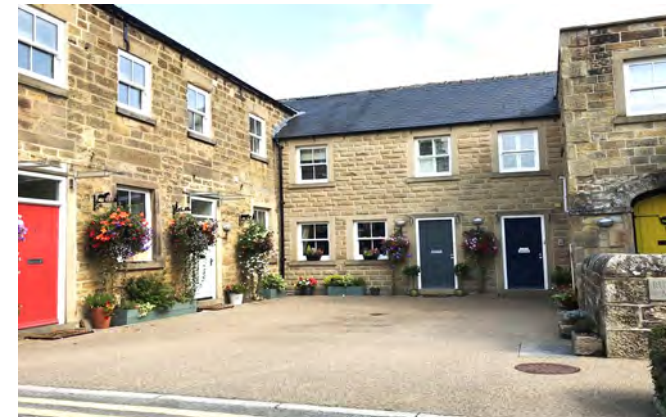
Individual painted doors in courtyard
